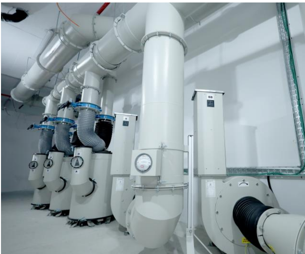
Filter bank – multifilter CBRN filtration unit
